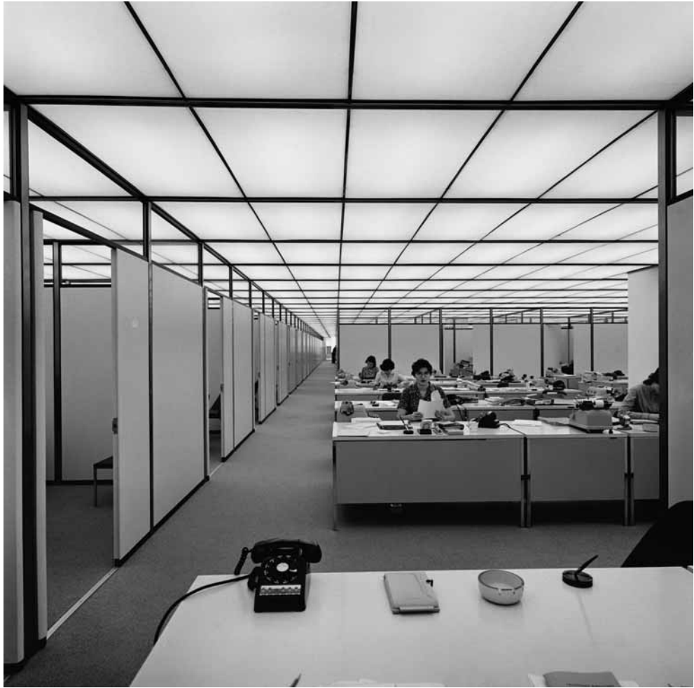
Skidmore Owings & Merrill (Natalie de Blois and Gordon Bunshaft, principal designers), Union Carbide Building, New York City, 1960, typical office interior.
