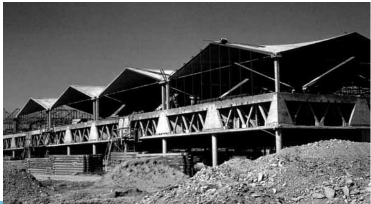
O'Neil Ford, Texas Instruments Semiconductor Building, Richardson, Texas, 1956–8, construction photograph.
